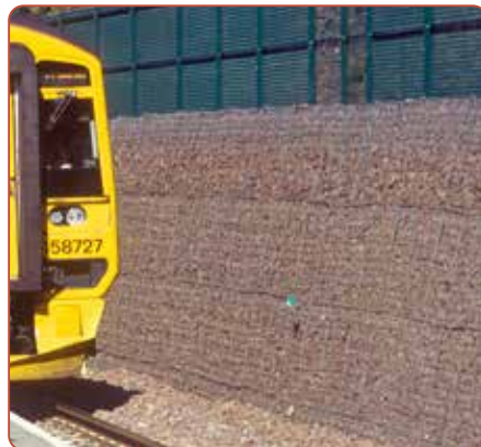
SSMP235 Gabion Cage Wall Prototype picture
